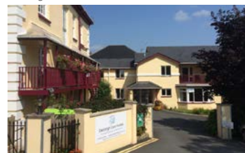
Eastleigh Care Homes, Periton Road, Minehead.
