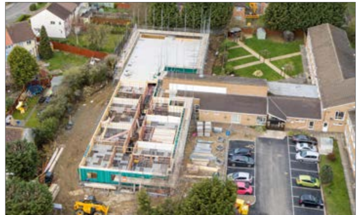
Ongoing construction of new 30 bed extension at Diamond.
